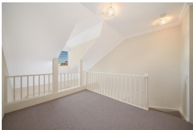
Figure 32 View inside Apartment 34/13 Earnest Place illustrating the dormer windows also provide solar access to the living room area below due to the mezzanine design
