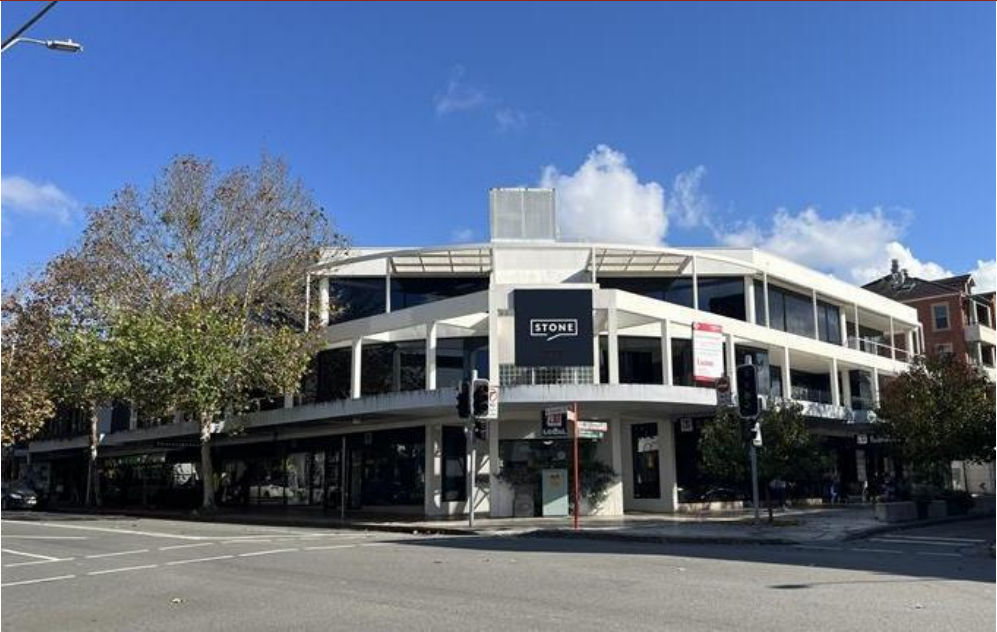
Figure 3 View of the site from corner of Alexander Street and Ernest Street
