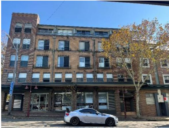
Figure 7 78-80 Alexander Street, adjacent to the site to the north
